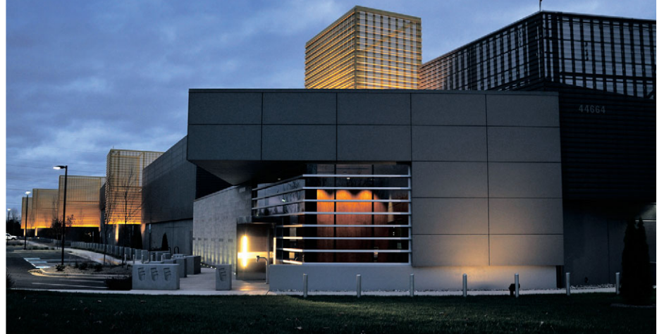
The RagingWire data center in Virginia.
